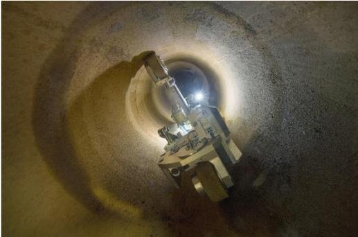
Following successful field trials, we have been using ULC Robotics' Cast Iron Joint Sealing Robot ('CISBOT') to fix, rather than replace, lengths of gas pipe in some of London's most high-profile locations. Our two major trials took place on Oxford Street and The Strand, and the success of these projects led to us deploying CISBOT on Park Lane, Regent Street and Covent Garden.
