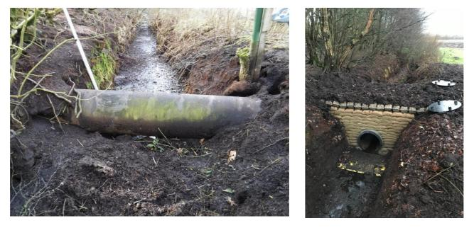
Figure 2: Protection of pipeline via construction of a culvert (before and after intervention)
