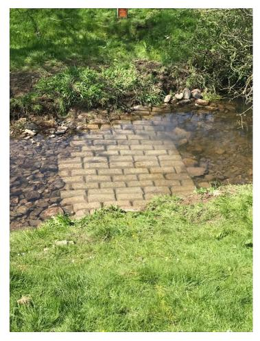
Figure 1: Ditch remediation using cobbled matting to protect the pipeline
