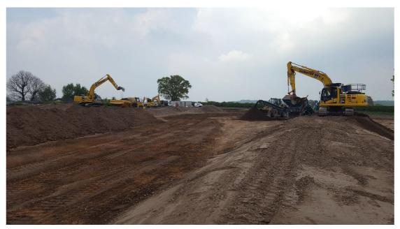
Figure 4: Pipeline protection via soil importation, New Farm, Redhill, EM Network
