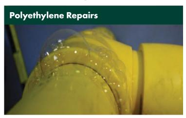
If a plastic pipe needs repairing, the only option for our repair teams is to cut out and replace that section of pipe.
