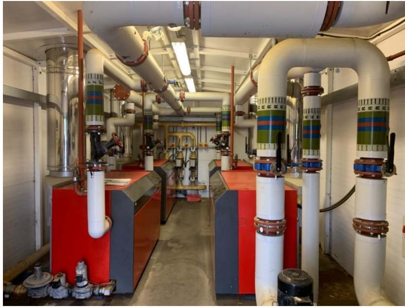
Figure 3 – modular boiler system.
