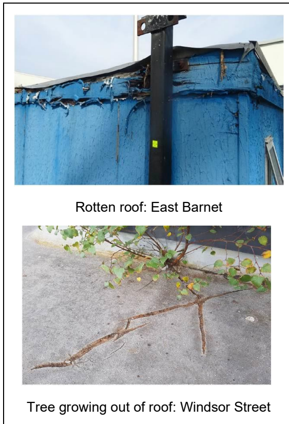
Figure 2: Problems with Roofing
