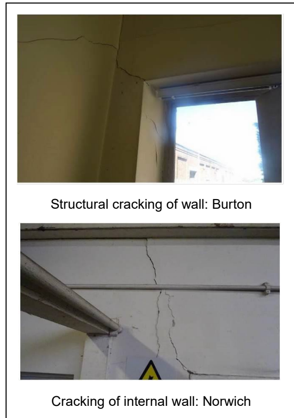
Figure 3: Structural deficiencies
