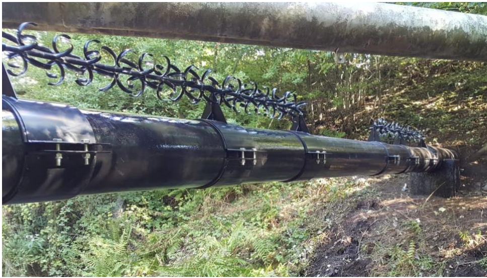
Figure A3: Example of Anti-climb rotational device
