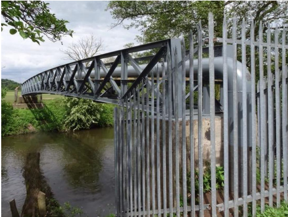
Figure A1: Example of Palisade Fencing
