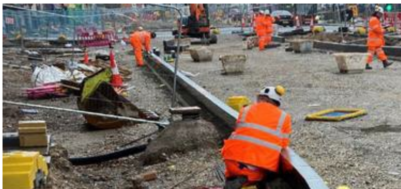
Figure 21: West Midlands team performing essential mains replacement works
