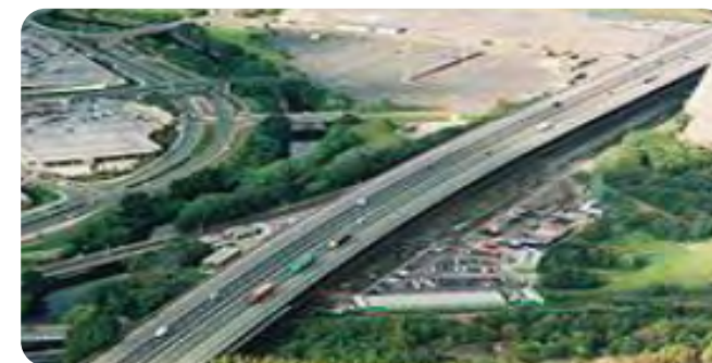
Tinsley viaduct (A2.4)
