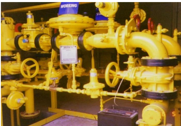
Figure 5: An example of a Twin stream Donkin 280, Donkin 305 'Active/Slam auxiliary controlled with Wafer check'
