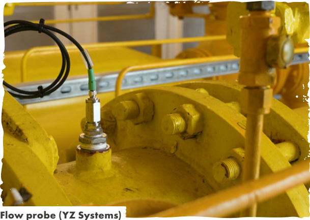
Flow probe (YZ Systems)
