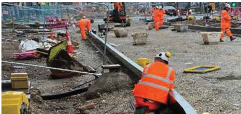
Figure 18: West Midlands team performing essential mains replacement works
