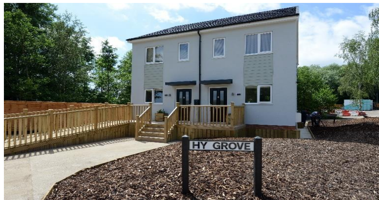
Figure 6: The UK's first homes with appliances entirely fuelled by Hydrogen
