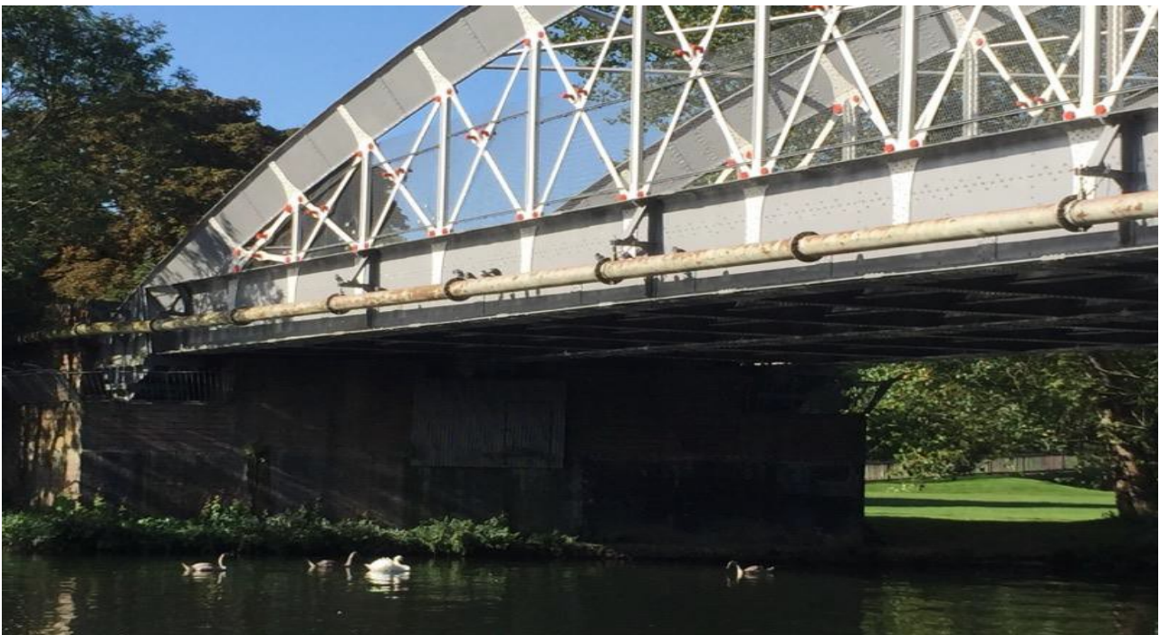
Figure 2: General view of main bridge span at crossing's north end
