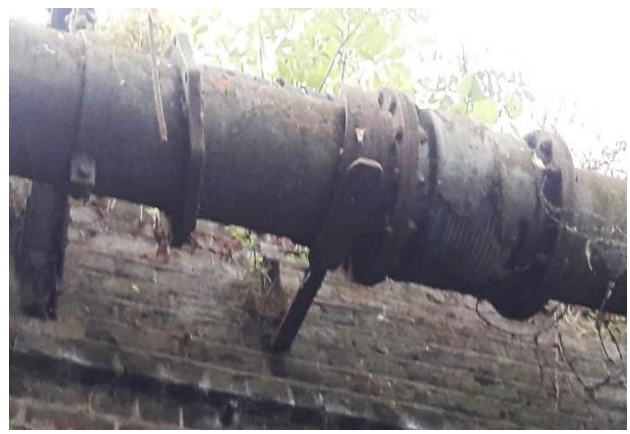
Figure 6: Expansion bellows, north side (left) & south side (right)
