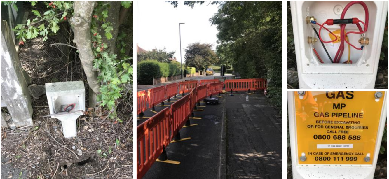
Figure 8: Test post installation before, during and after
