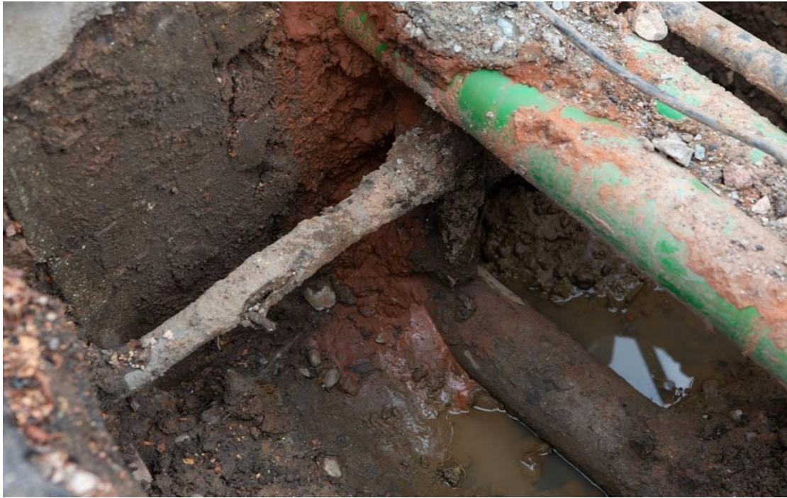
Cast iron main and service tee
