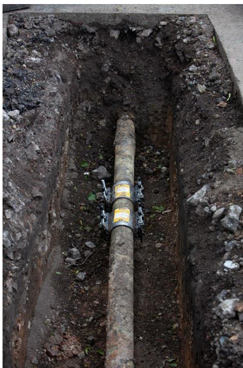
Picture 4: Example of a Main with Repair Clamps
