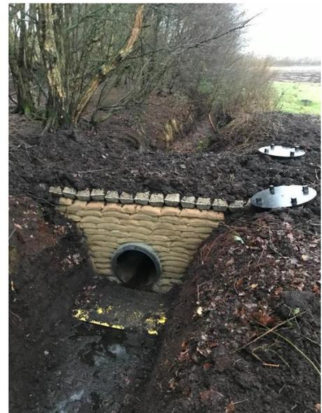
*Figure 2: Protection of pipeline via construction of a culvert (before and after intervention)*
