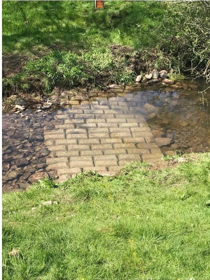
*Figure 1: Ditch remediation using cobbled matting to protect the pipeline*
