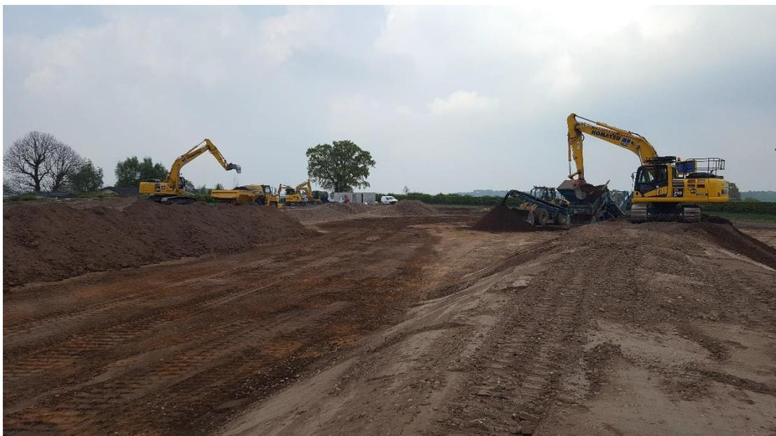
Figure 4: Pipeline protection via soil importation, New Farm, Redhill, EM Network
