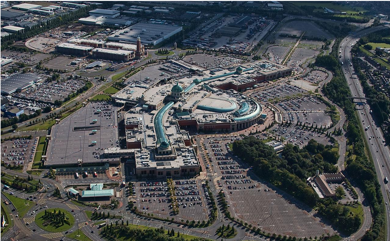
Figure 12: Example CDS Supply – Trafford Centre (by CB)
